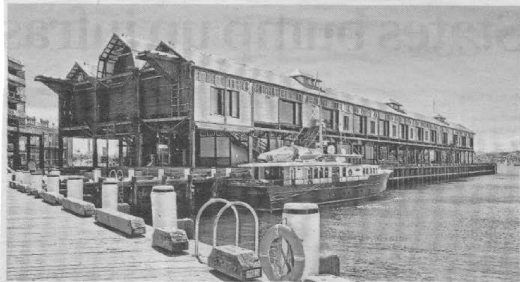
Pier 8 & 9 at Walsh Bay is expected to attract keen interest.
